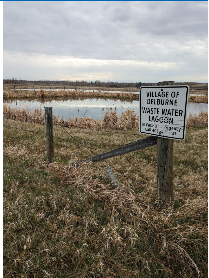
Delburne's lagoon system was constructed and upgraded from 1979 to 1984. It is located East of the Village and has 7 cells.
